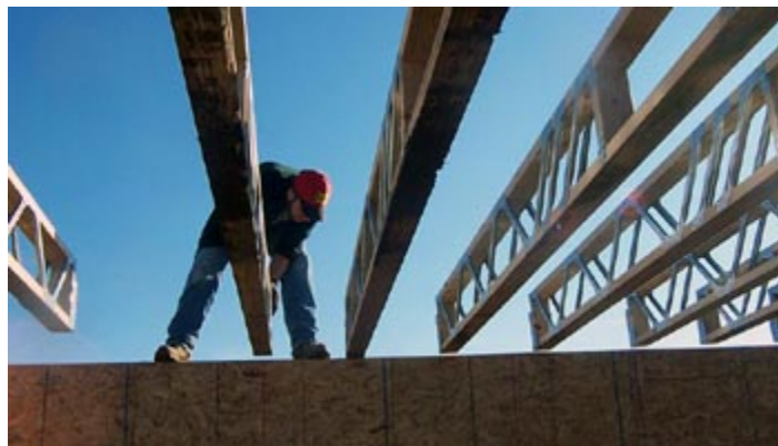
Wood top and bottom chord/open metal web truss floor joists Photo Courtesy Earthen Concepts & Developing
