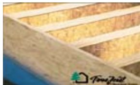
Trus Joist® and engineered lumber rim joist floor framing Photo Courtesy of Weyerhaeuser
