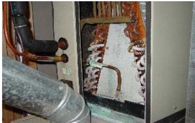
**Go back to the exterior unit and to determine if the suction line is sweating and cold to the touch and if the liquid line is warm to the touch. Frost or ice on the suction line indicates a problem and may be due to an air handler blower speed problem, a dirty filter, an obstructed evaporator coil, a defective metering device, low refrigerant charge, or other conditions.**
